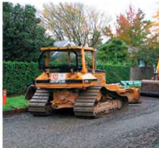
Prepared subgrade for 20,000 sf (2000 m 2 ) Portland, OR street retrofit with PICP
