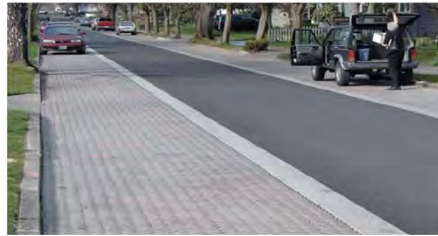
Portland, OR street project with PICP parking lanes
