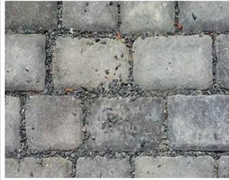
Green Alley Pavers
