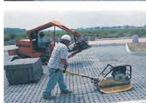
Aggregate base is spread and compacted; pavers are delivered ready to install. After placement of bedding course, joints and/or openings are filled with small aggregate and the pavers are compacted. Joints may be filled mechanically as shown.
